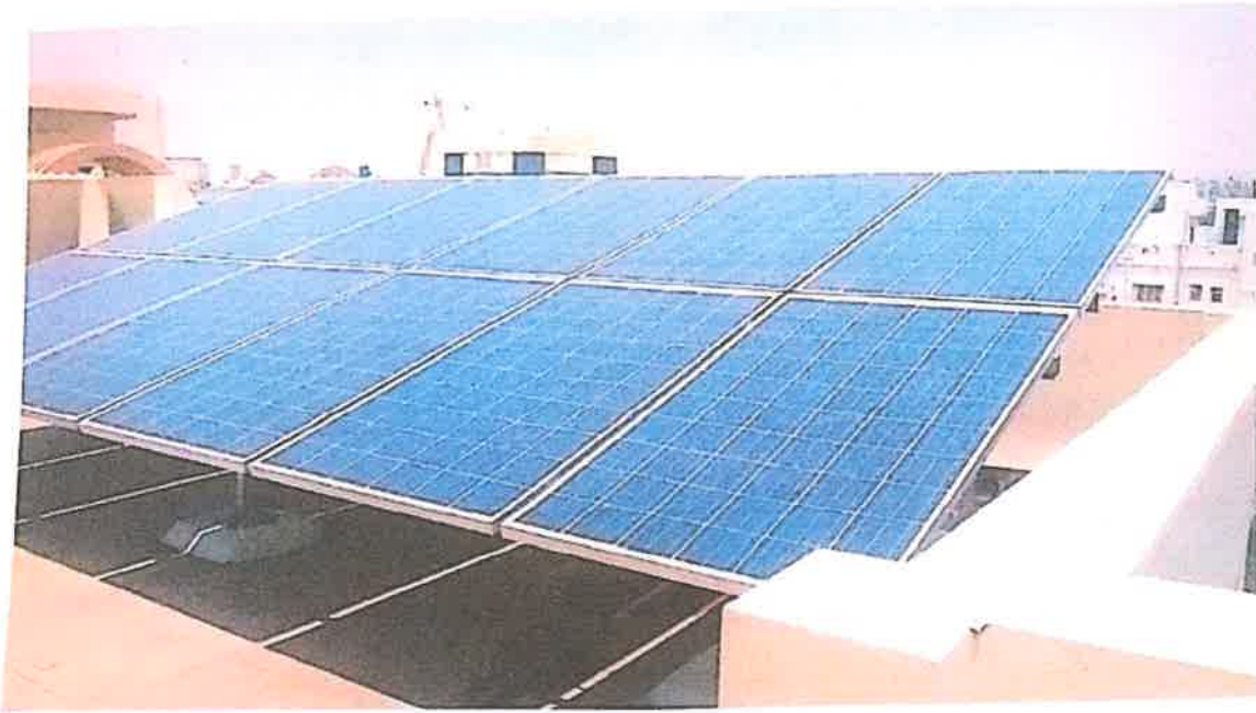
5KW on GRIDTIE SOLAR SYSTEM
