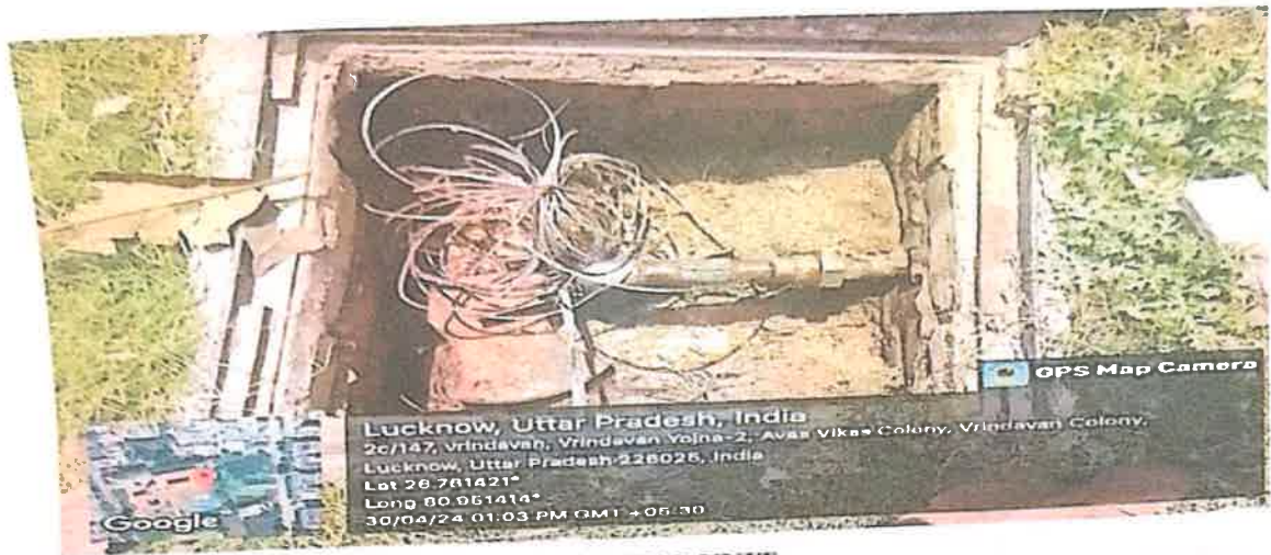
WATER BORING UNIT
